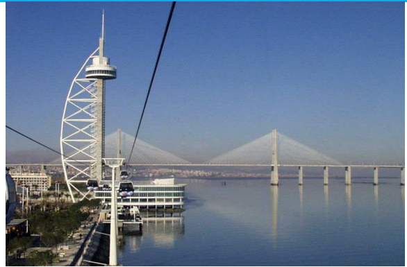
Vasco da Gama tower and bridge
